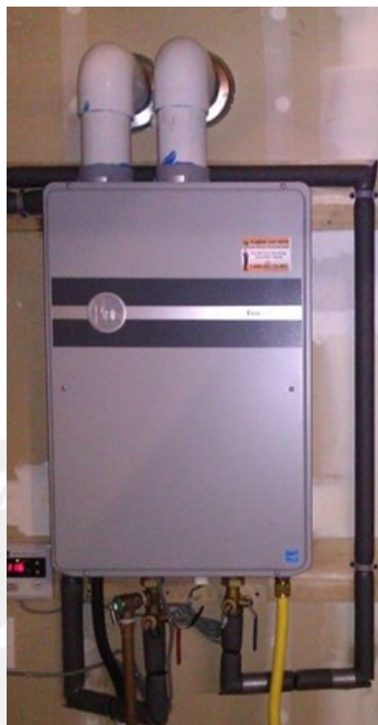
Here are two photos of the equipment that was installed at the Golden Key Apartments in Jackson. Rheem Tankless water heaters (left) and Lennox HVAC equipment (right), which are both extremely efficient pieces of equipment. Each can be PVC vented as well which cuts down on install costs.
