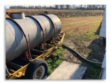
The referenced church uses an old agricultural tank for holding water that is delivered to the tank on occasion. The tank is positioned behind the church and is connected to an electric mechanical pump that can be activated to pump water to the church when needed for bathroom and other purposes. The on-site well failed and is inoperable.
