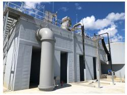
Wastewater enters the facility in the large pipe to the left. This structure contains a series of grates, screens and other equipment to remove plastics, metals, glass, grit and other solids that wind up in wastewater.
