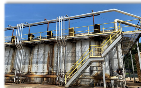
By insulating their piping network, temperatures were more consistent, heat loss was reduced by more than half, which in turn greatly reduced the load on the facility's boilers.
