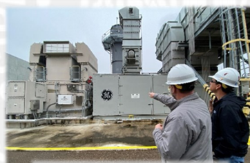
Discussing the GE "black start" combustion turbine and generator
