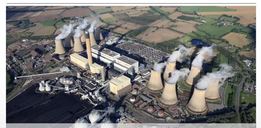
2 of 6 units fully converted to biomass, 3rd unit at 90% biomass
